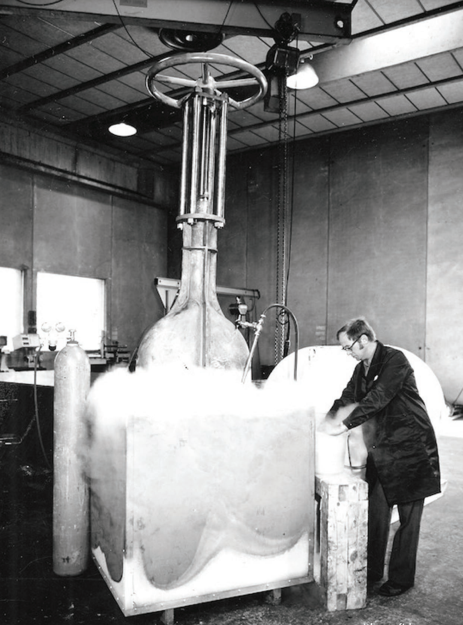
Cryogenic testing of a Westad gate valve for LNG in the late 1960s.
